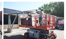
Attach braces, beams and purlins
