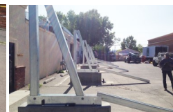
Install foundations at correct intervals
