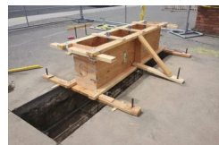
Excavate and form foundations
